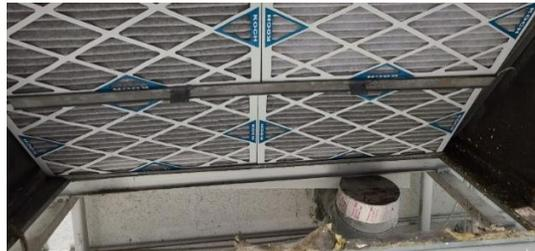
High-efficiency filters such as HEPA, can trap some virus particles, however ventilation systems are designed to use specific types of filters. Installing a higher rated filter can result in the necessity to change or even replace the ventilation system. Changing the system would still require a number of air passes through the ventilation system before the system was effective.
